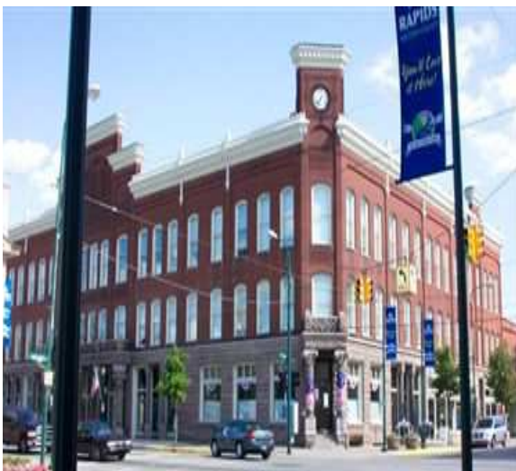
The Nisbett Building
