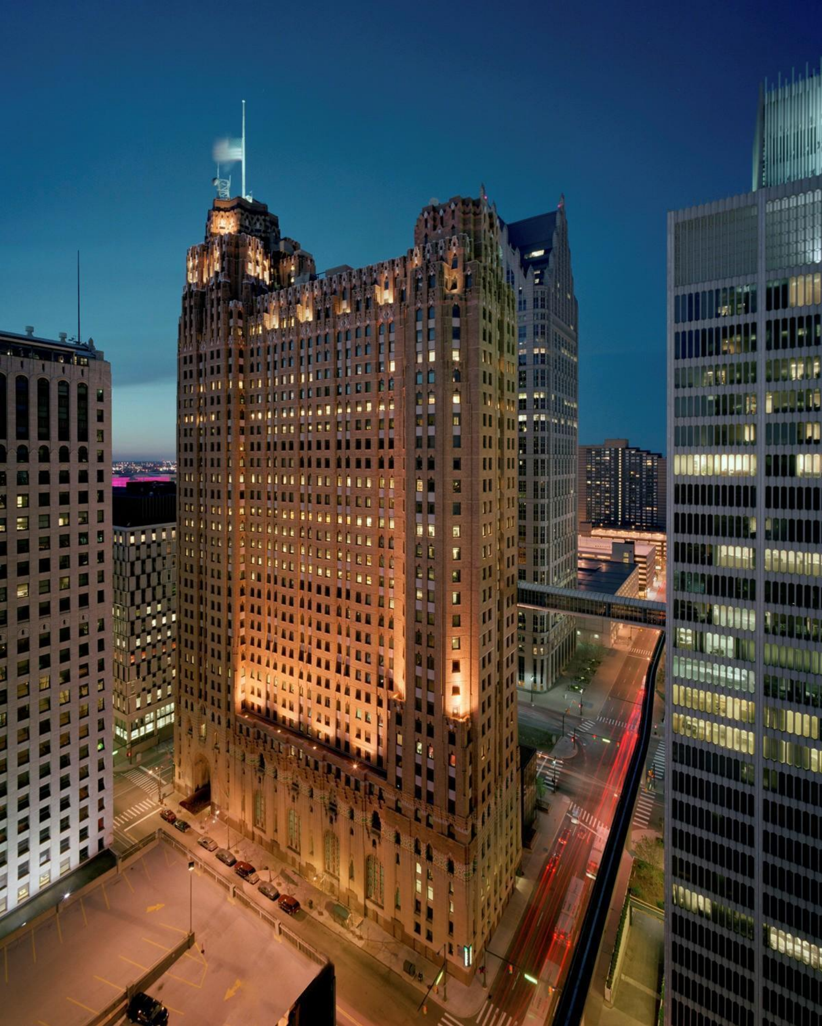
1929 Guardian Building, renovation complete. From the session, "Restoring a National Landmark – Detroit's Guardian Building," presented Friday, May 16, 2:15 PM - 3:30 PM. CREDIT: SmithGroup
