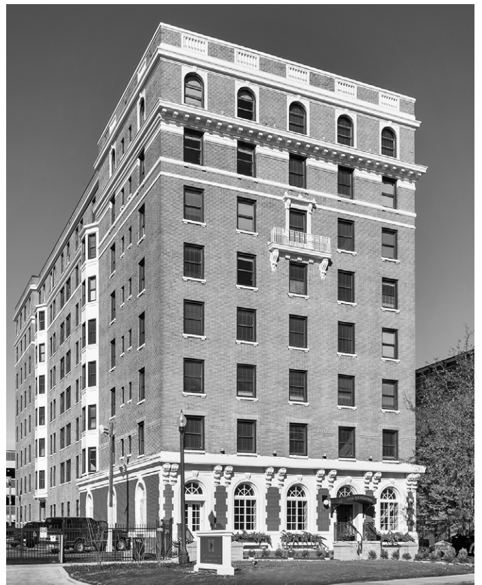
The Hamilton Apartments Rehabilitation, Detroit, Michigan. Photo by Hamilton Anderson Associates.
