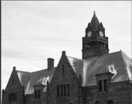
CITY HALL, Bay City, MI Clay Tile Roofing & Copper Work
