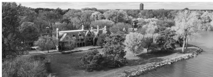
Ford House Main Residence Lakeside Aerial, Grosse Pointe Shores. Photo by FORD HOUSE.
