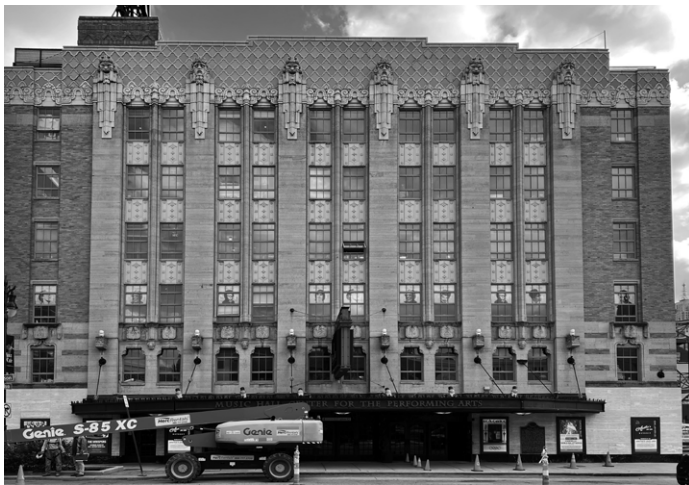
Music Hall, Detroit, Michigan. Photo by John P. Biggar. Submitted by Integrity Building Group.
